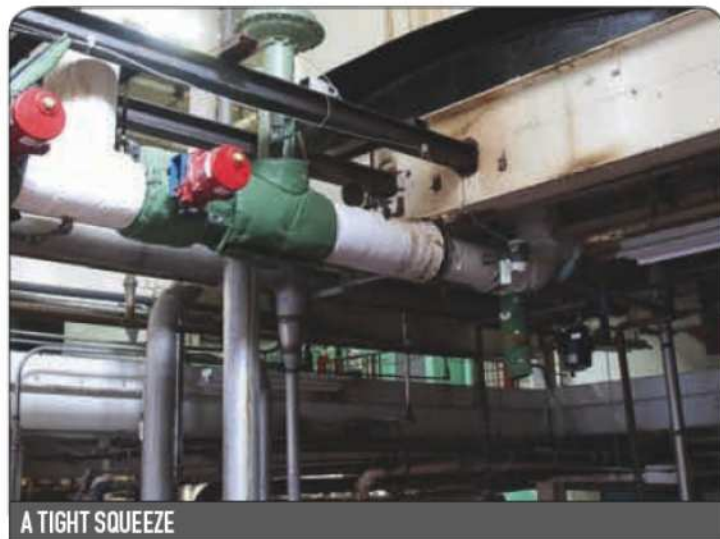
Figure 5. Matt chose the Swirl meter because its piping geometry left little room for straight-run piping to condition the steam flow.
